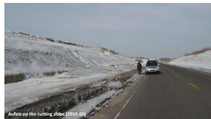
Aufeis on the cutting slope (2010.03)
